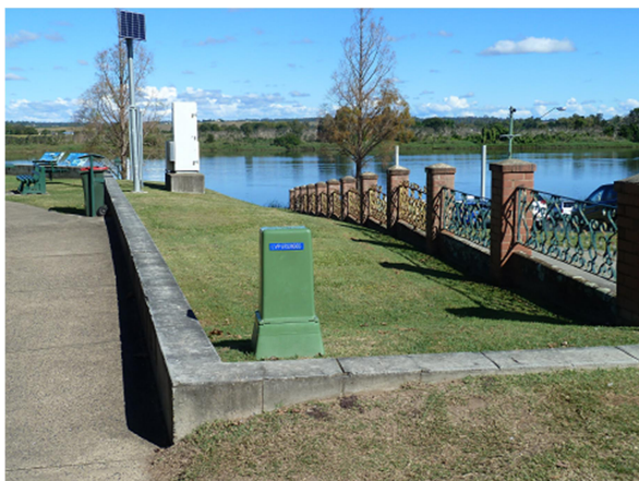
Masonry block levee wall adjoining Prince Street
