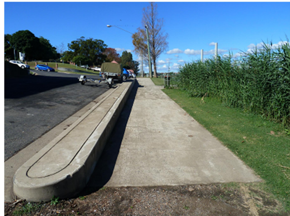
Concrete path, kerbing and road pavement
