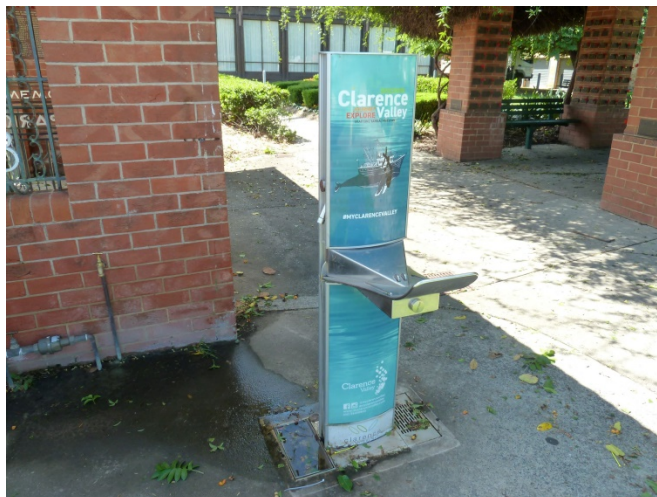
Figure 4.22: Water from drinking water fountain pools at base of entry gate brick work
